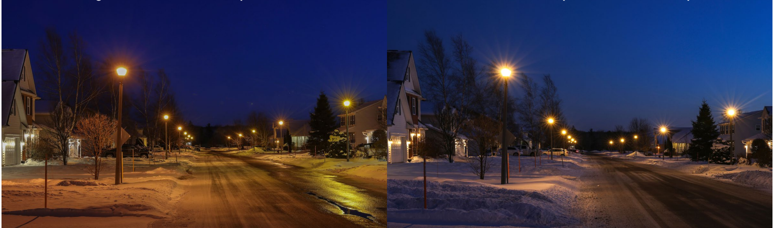
Before: 100W High Pressure Sodium HID Lamps
